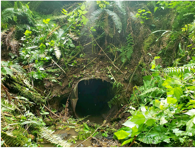
Culvert Removal, Before
